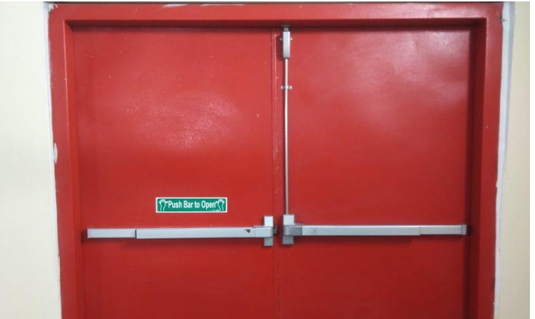
Emergency Fire Exit Door
