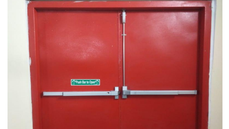
Emergency Fire Exit Door
