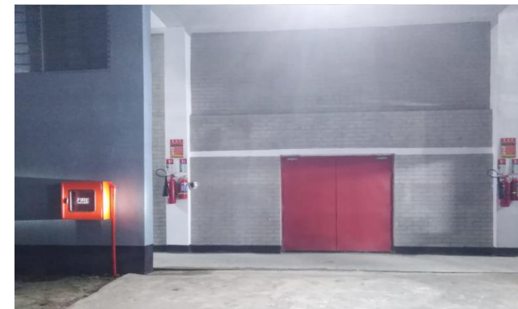
Fire Exit Door
